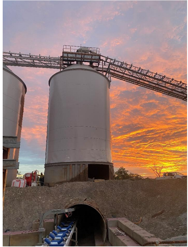
Figure 7: Mineral Hill Plant refurbishment includes – crushers & ROM bin, conveyors, fine ore bins & feeder tunnels, mills & grinding circuit, flotation plant, electrical network and supply, water supply, reagent dosing, safety equipment, instrumentation, pumps and piping.
