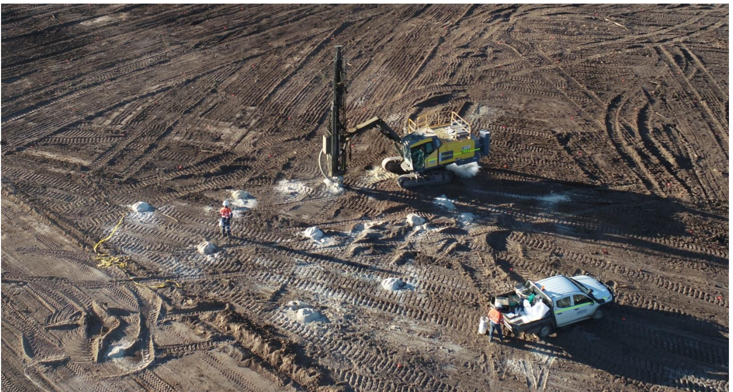
Figure 2: Pearse North open pit drilling is underway.
