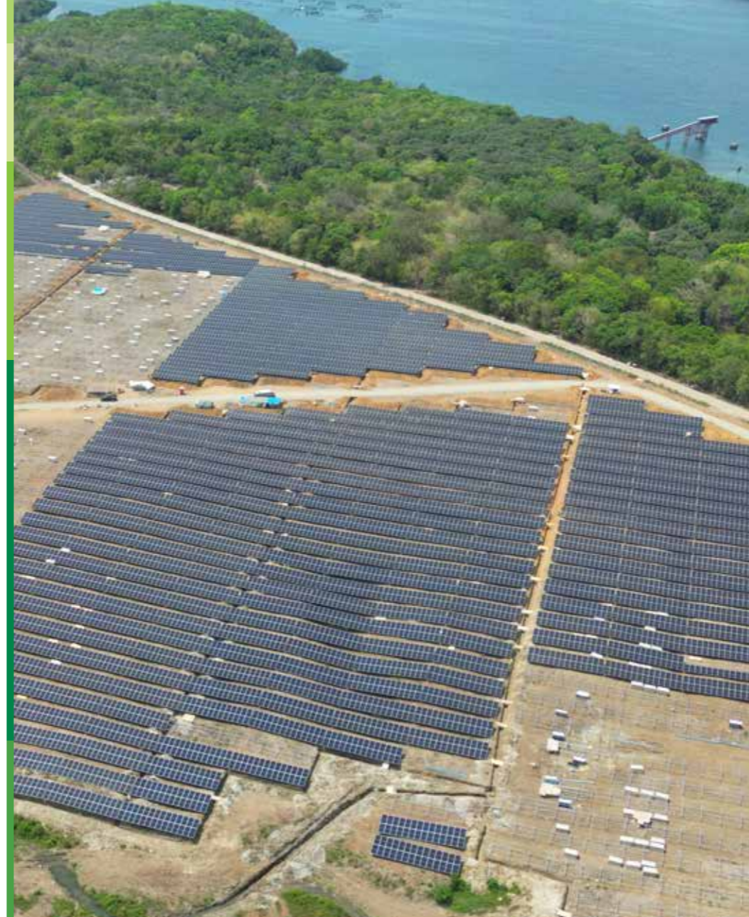
The 75MW Palauig Solar Power Plant under construction in the Philippines
