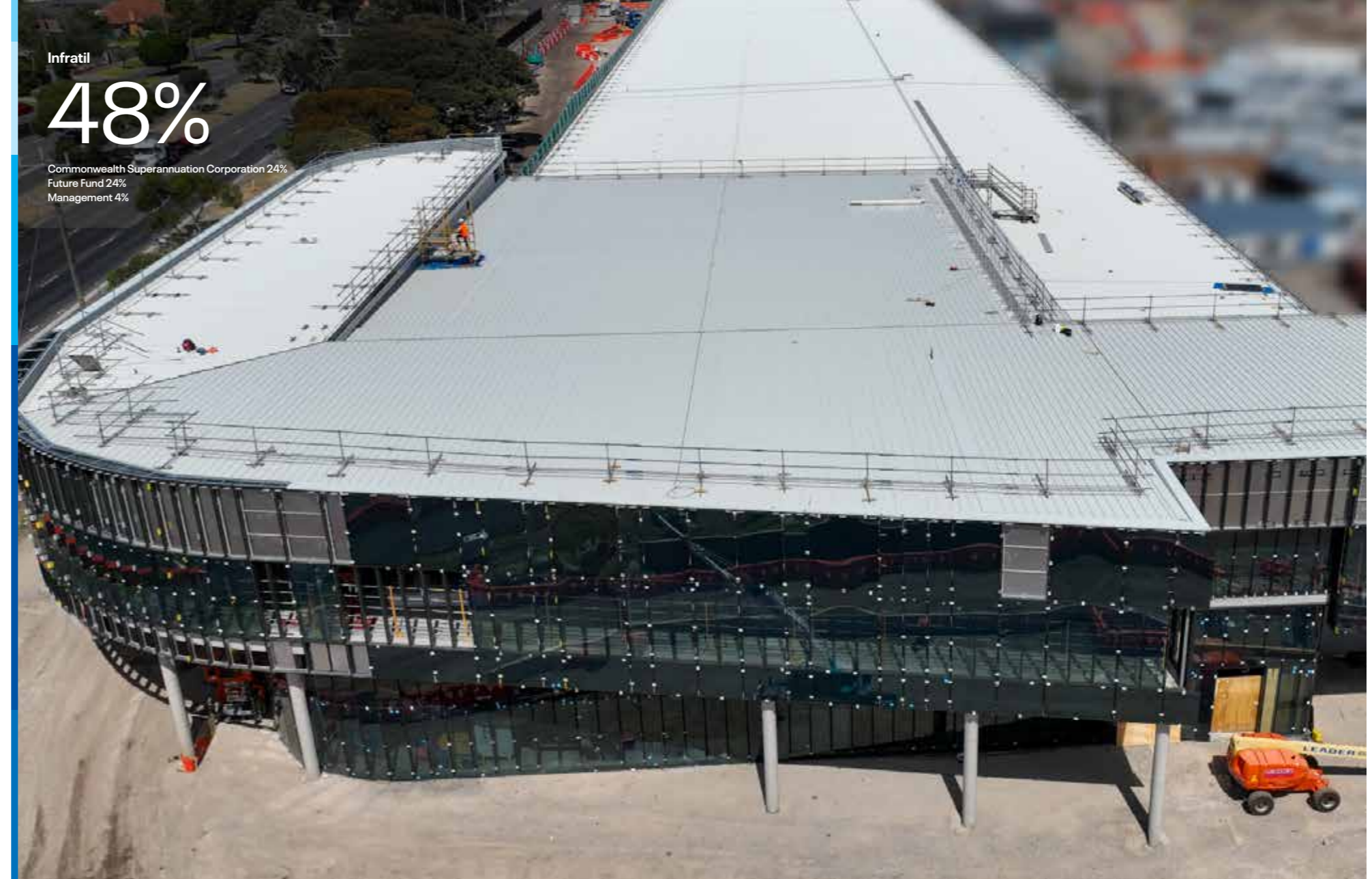
Brooklyn 1 under construction in Melbourne
