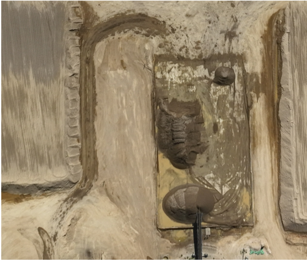
Image 1: Wet concentrate overflow storage pad. Used for >12% moisture for free draining of water. Status: 17 th May, Complete.
