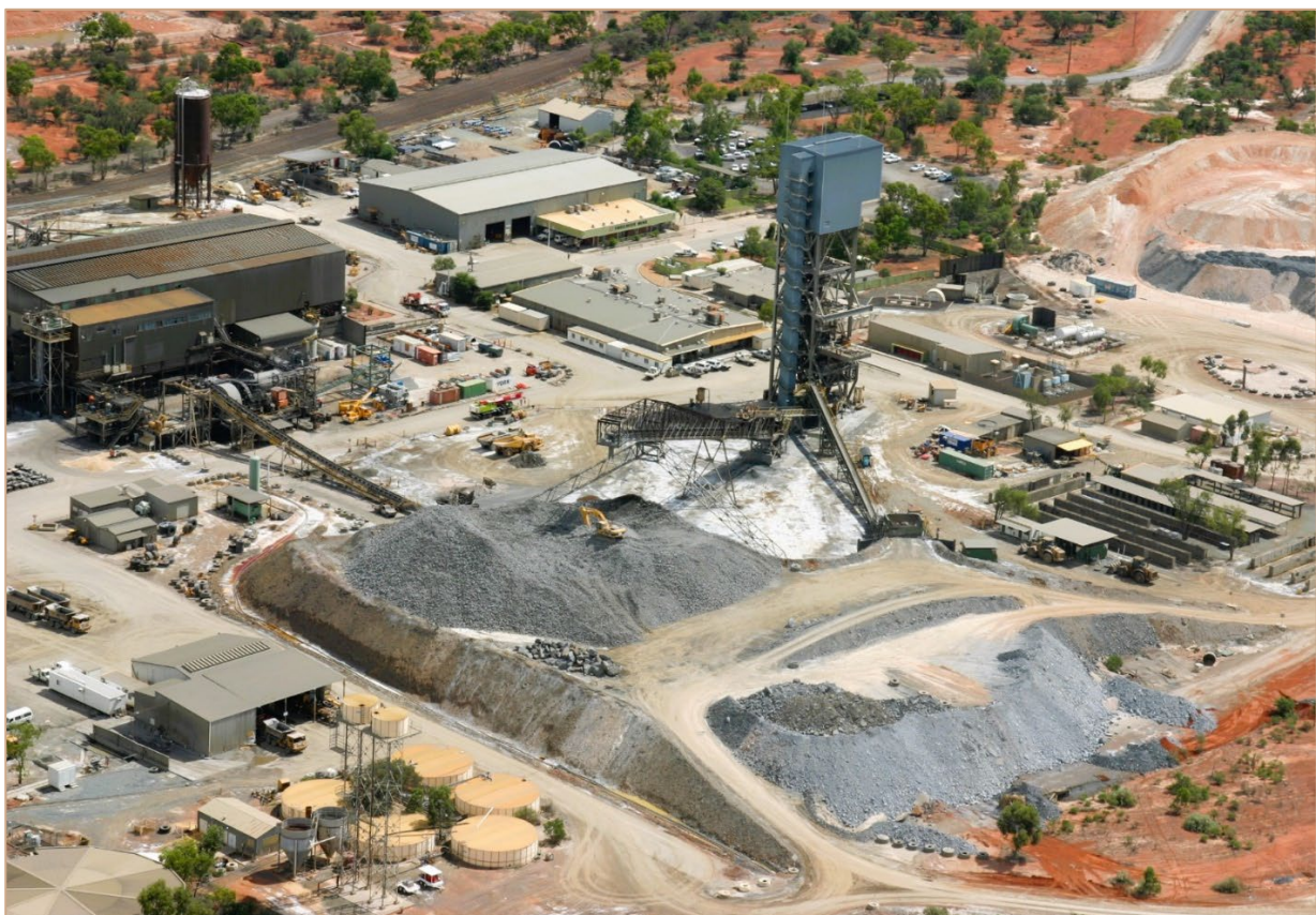
Endeavor Mine, Cobar NSW, Australia
