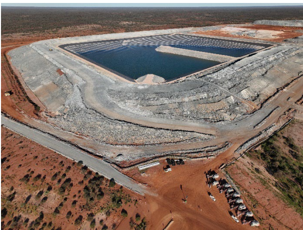
Figure 7: Tailings Storage Facility (TSF) Cell 1
