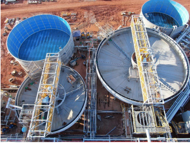
Figure 14: Process and Tails thickeners
