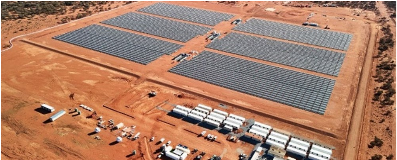
Figure 22: Aerial photograph of the ~31,000 solar panel farm and temporary construction camp
