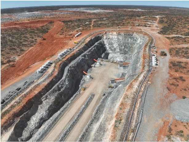
Figure 3: Portals at Mt Mann box cut
