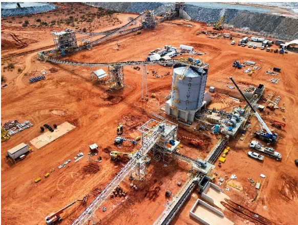
Figure 9: Dry plant commissioning commenced late March
