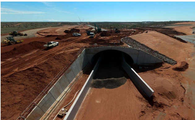
Haul road at Warrirda/Onslow Rd overpass
