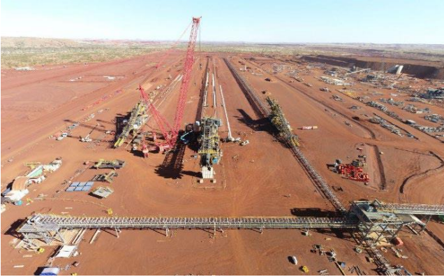
Stacker and reclaimer assembly ongoing
