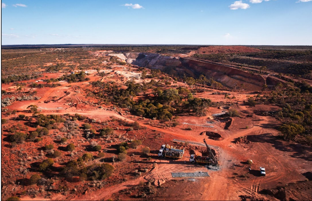
Diamond and RC Rigs drilling underground and resource targeted holes at Orion Pit
