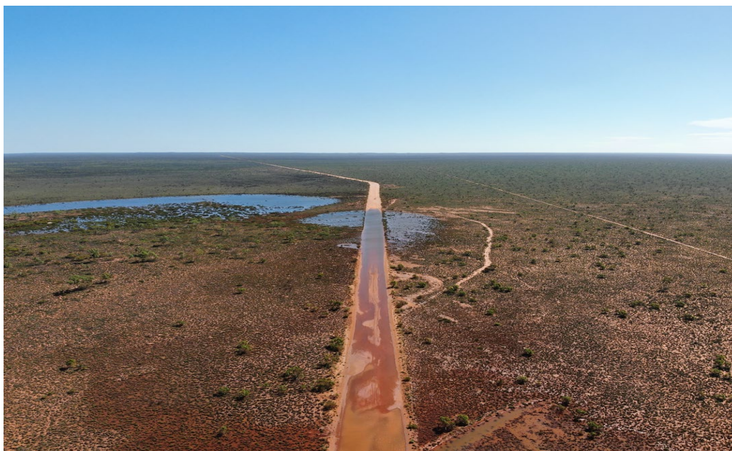
Figure 1: Great Central Road Flooding 20 March 2024
