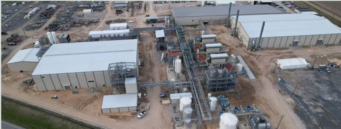
◀ Vidalia AAM facility
