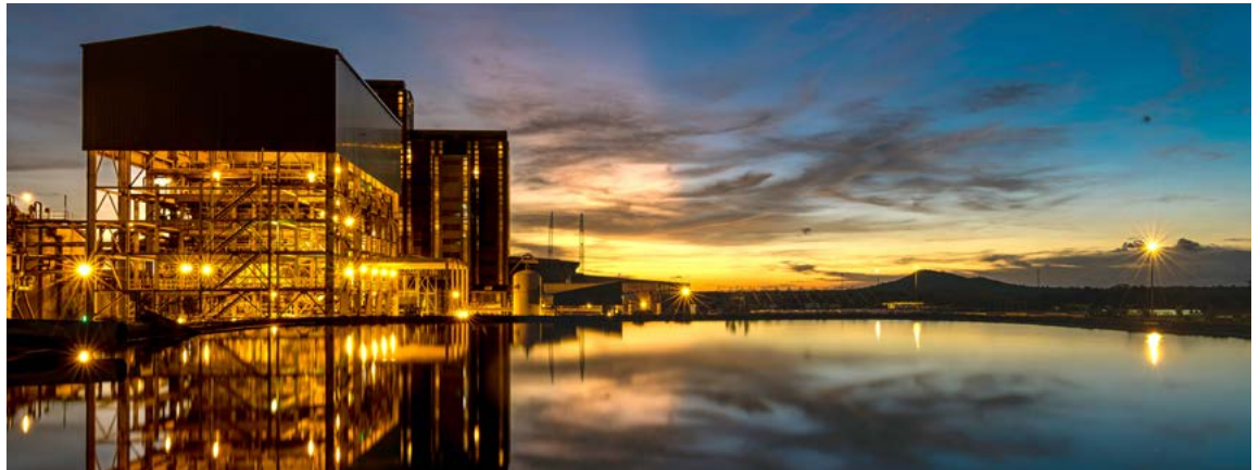
Balama processing plant
