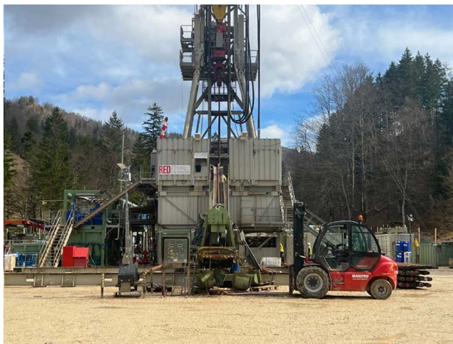
The RED Drilling & Services GmbH (RED) E200 drill rig drilling at Welchau
