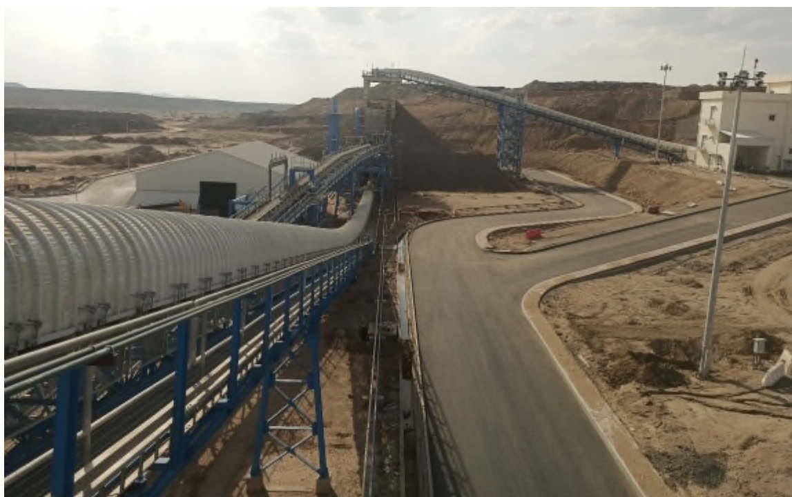
Image: Crushed Copper Ore Stockpile and Mill Feed
