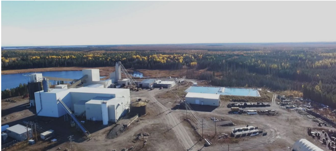
Figure 6: Wabowden Project - Bucko Mine and Processing Facility
