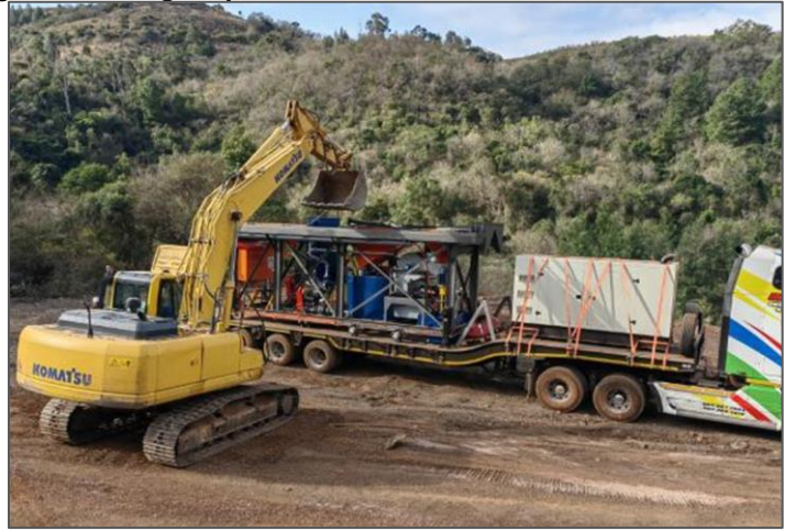
Figure 11: DMS being offloaded on site.
