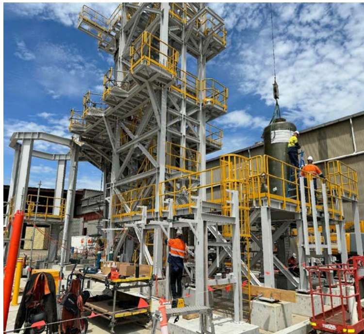
Spray Roaster mechanical equipment installation progressing
