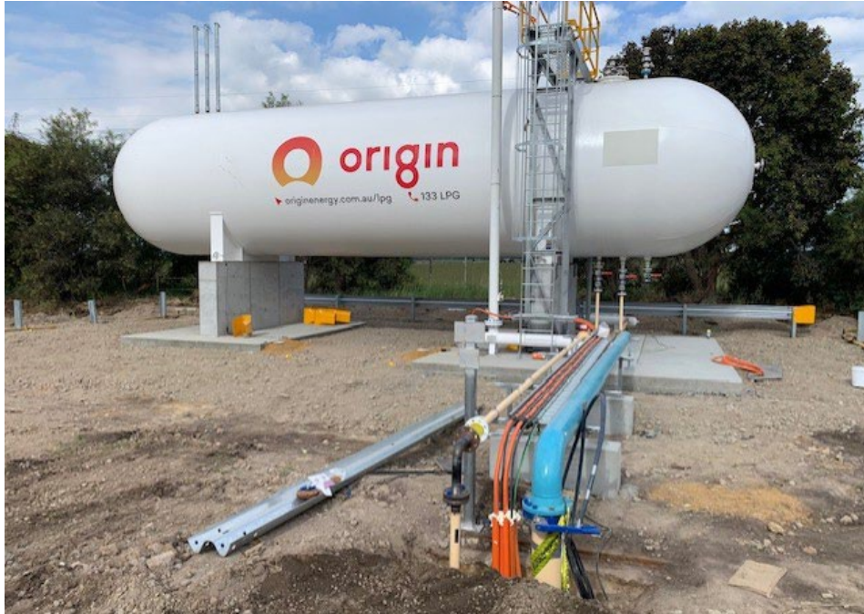
Origin LPG bullet and underground pipeline being installed
