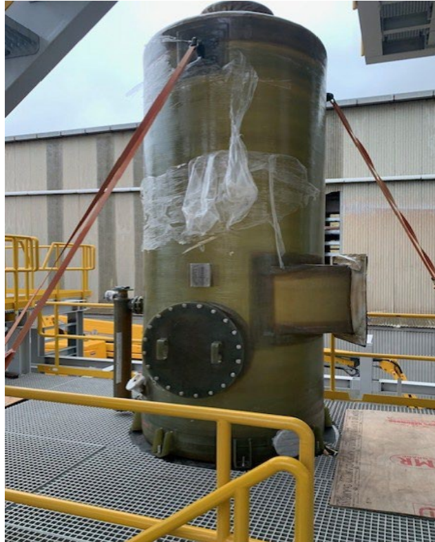
Spray Roaster tanks installed in final position
