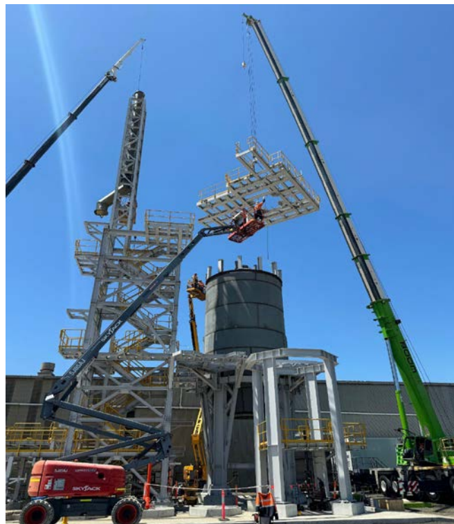
Installation of modularised Spray Roaster structural steel platforms
