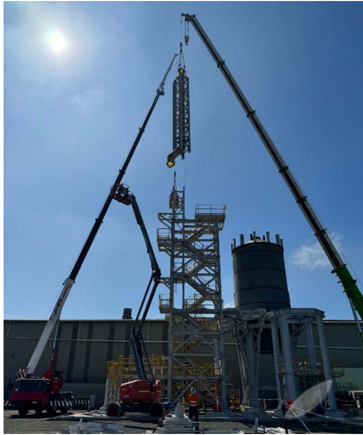
Installation of modularised Spray Roaster Stack structural steel with piping
