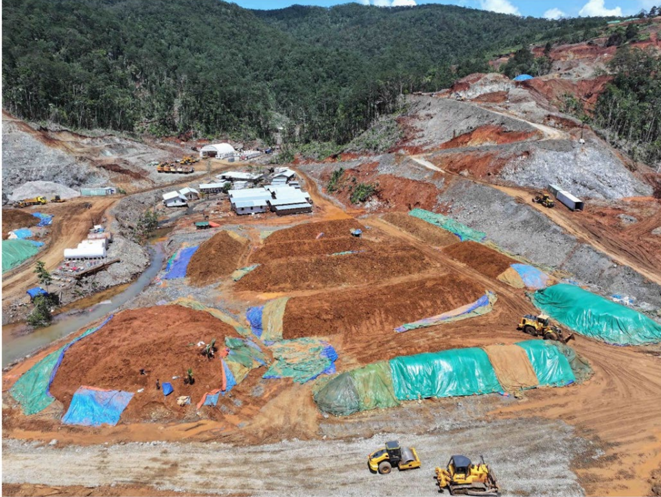
Photo 1 – Kolosori Project Site and stockpiles located near to the Kolosori Wharf
