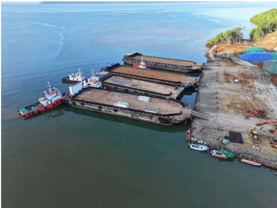
Photo 2 – Barges docked at Kolosori Wharf for barging of ore to a geared transport ship
