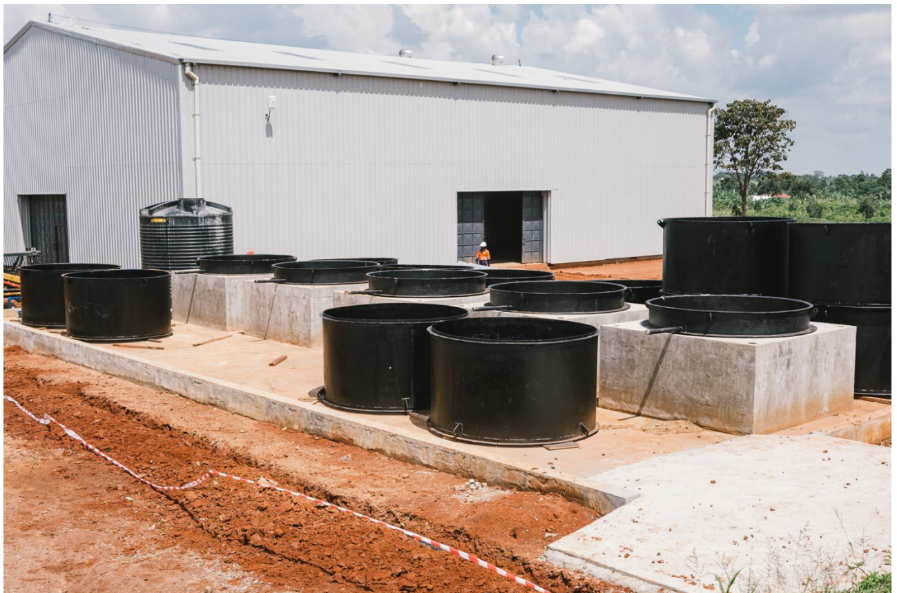
Figure 5: Crib shells which were being assembled for commissioning.
