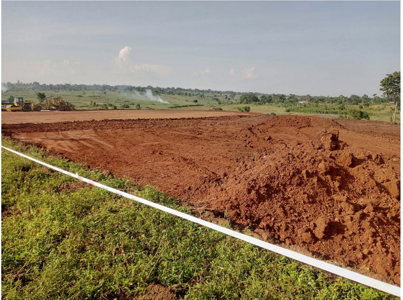
Figure 2: Removal of the topsoil layer across the Demonstration Plant facility area.
