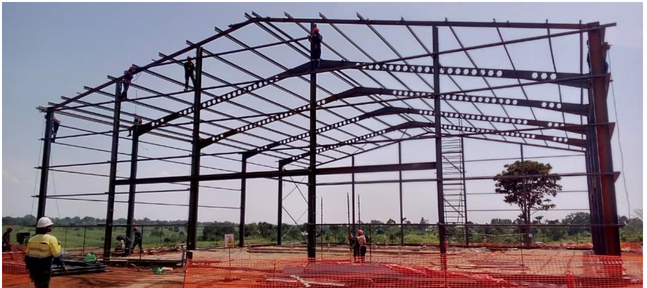
Figure 3: Makuutu Technical Facility frame structure erected.
