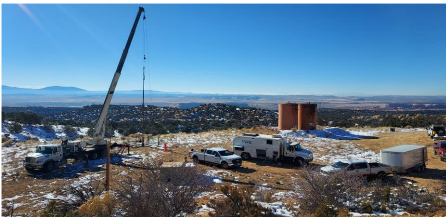
Figure 2: Wireline unit conducting brine sampling operations at Big Indian #1
