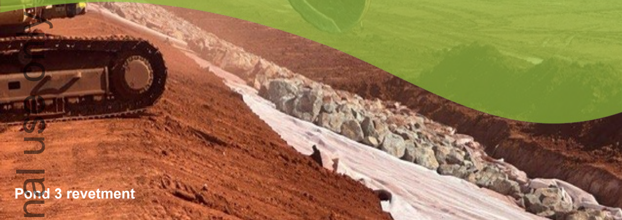
Pond 3 rock armour placement
