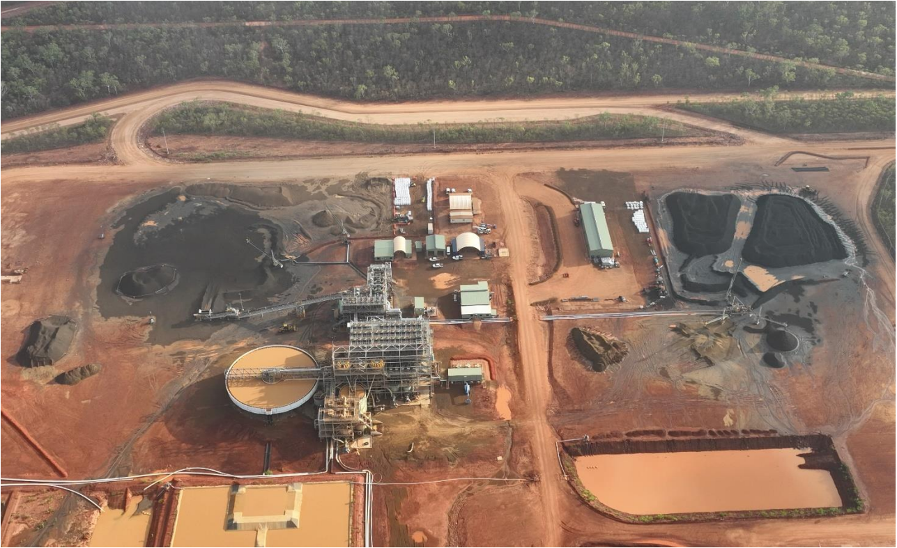
Figure 2: Thunderbird Process Plant site including Heavy Mineral Concentrate and product stockpiles (January 2024)
