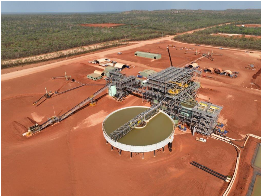
Figure 1: Thunderbird Process Plant site
