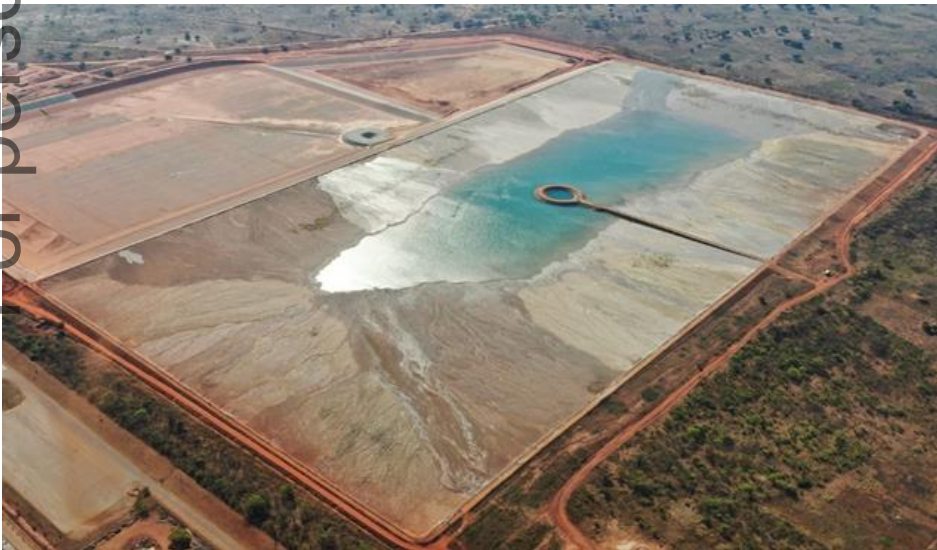
Tailings storage facility (cells 1 & 2)
