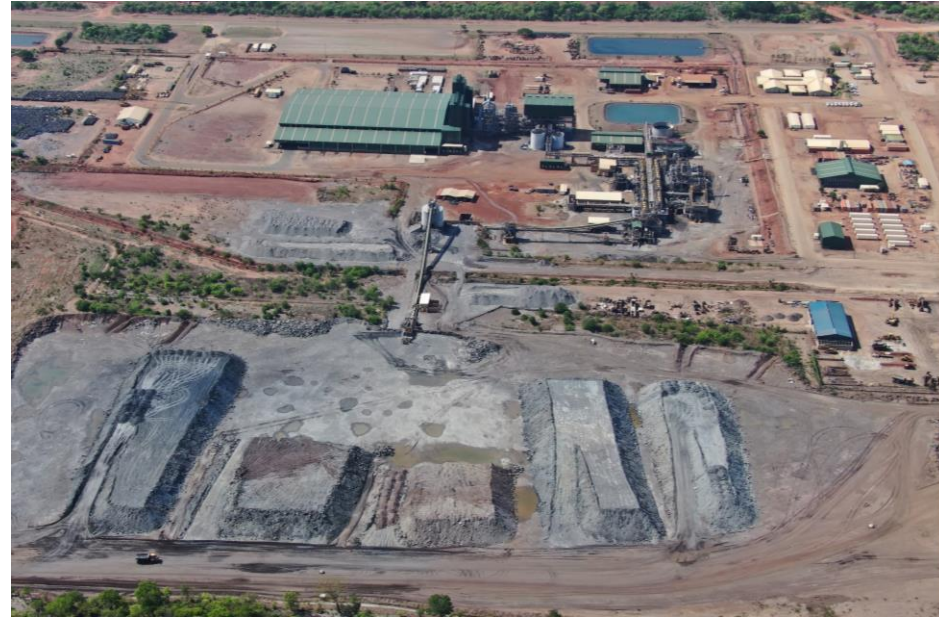
Process plant, product warehouse and ROM stockpiles
