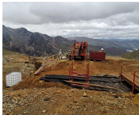
Image 3 Drill Pad Preparation
