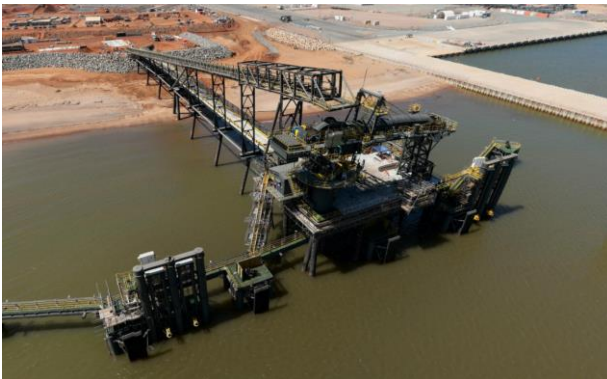
Transhipping wharf at Port of Ashburton
