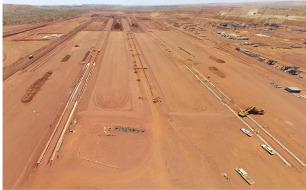
Stacker works and stockyard earthworks
