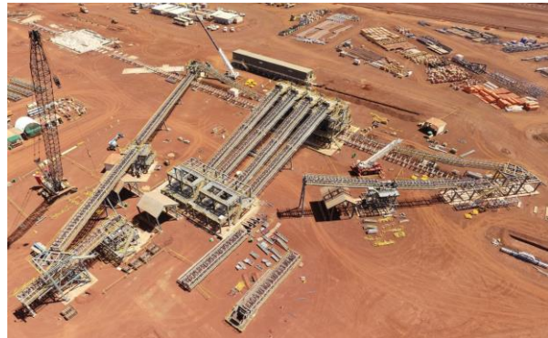
Ken's Bore crushing plant works
