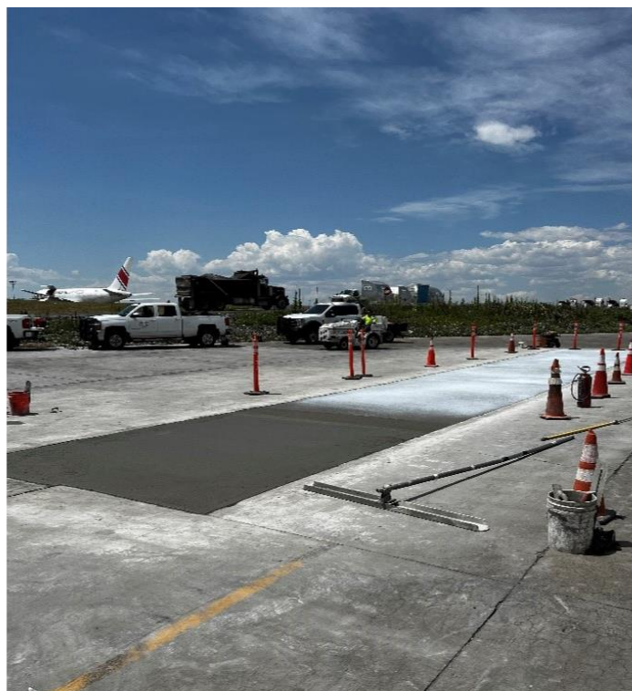
Figure 5. Full depth concrete panel replacement at Denver International airport
