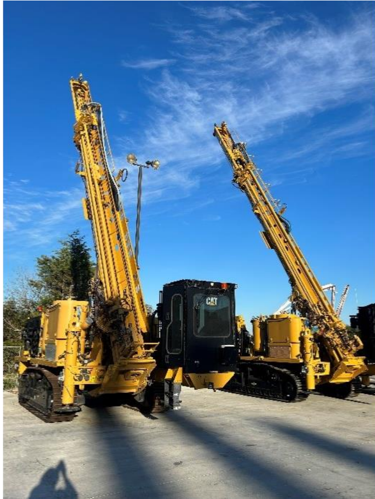
Figure 9. Drill Rigs test slab in use
