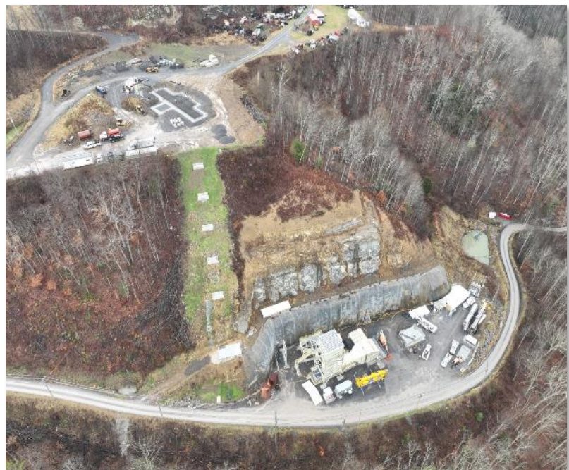
Image: Infrastructure works on the 2 nd VAM unit at Vent Shaft 18
