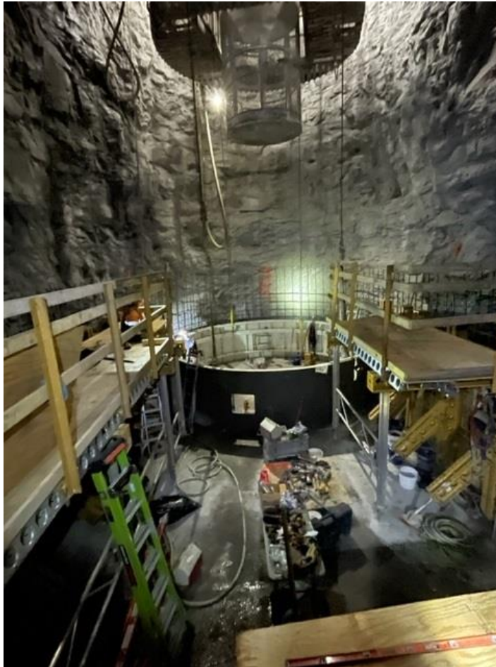
Image: Underground excavation works on the production hoist at Buchanan
