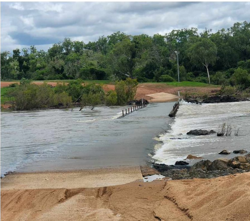
Walsh River crossing near Tartana Plant at 12 January 2024
