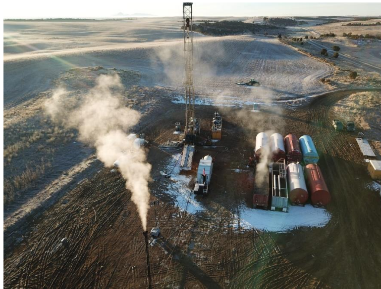
Figure 2: Jesse-1A well-site with flare-stack venting reservoir gas and helium to surface during flow-testing
