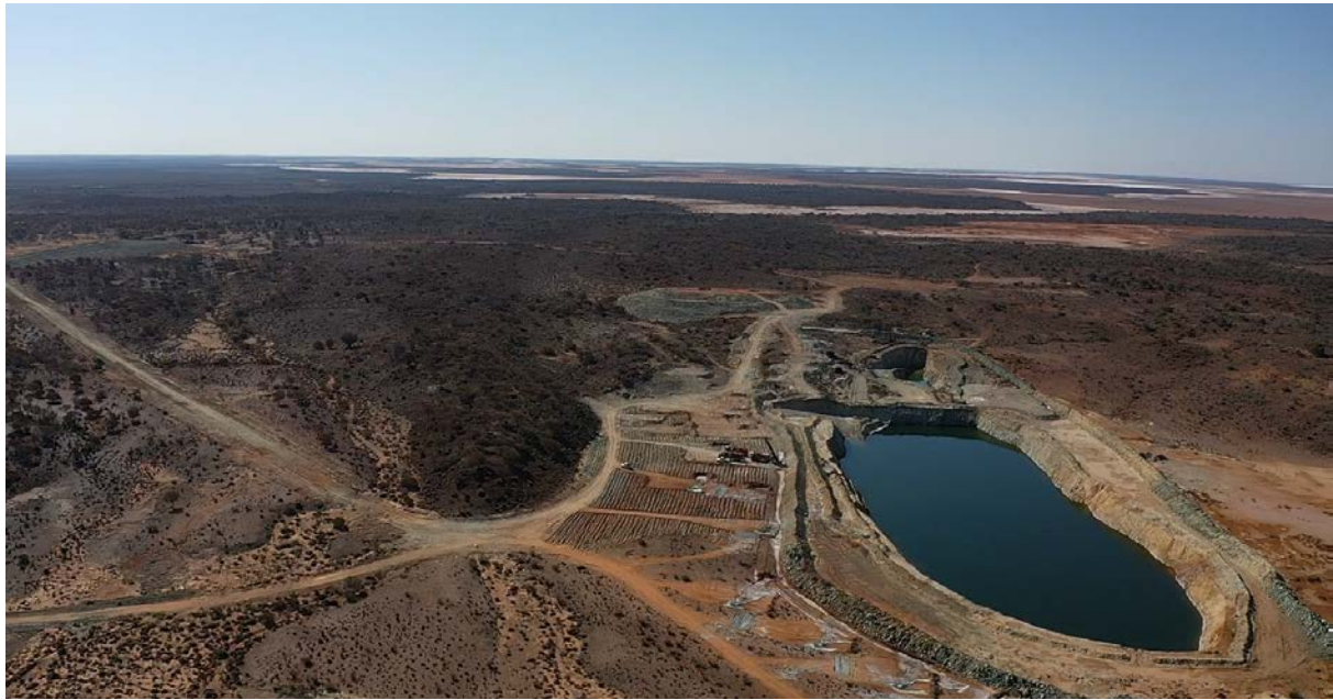
Figure 3: Devon Open Pit Gold Mine looking north towards Red October and Sunrise Dam
