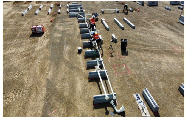
Figure 2: Mechanical crews commencing plant construction
