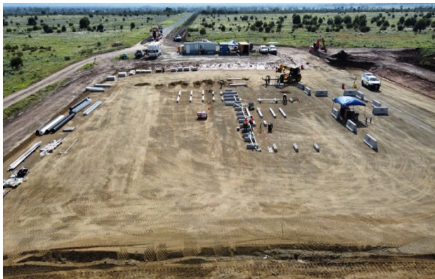
Figure 1: Completed CNG Facility pad
