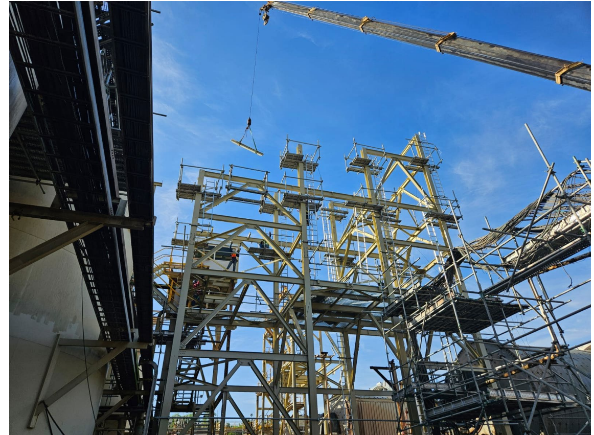
Progress shot of the Plant #1 grinding circuit being replaced
