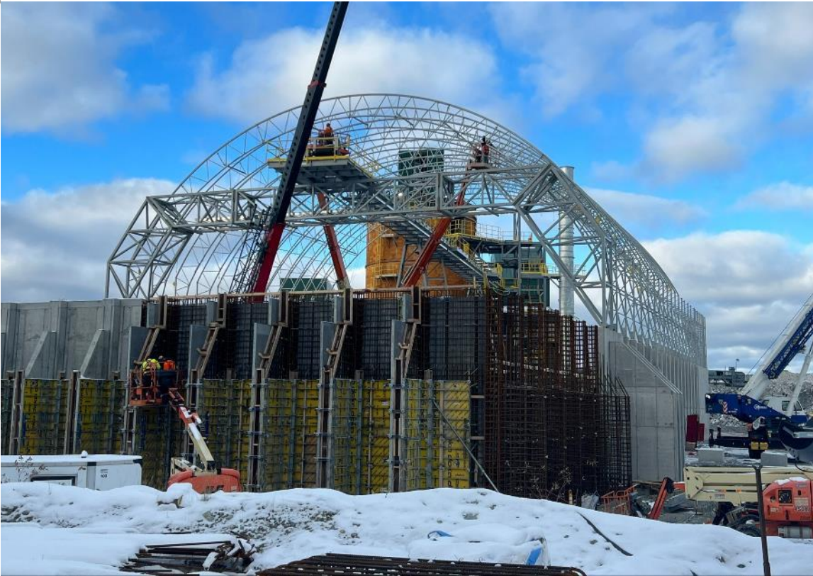
Crushed Ore Dome construction
