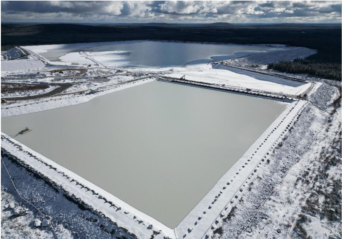
Tailings Storage Facility 1 project
