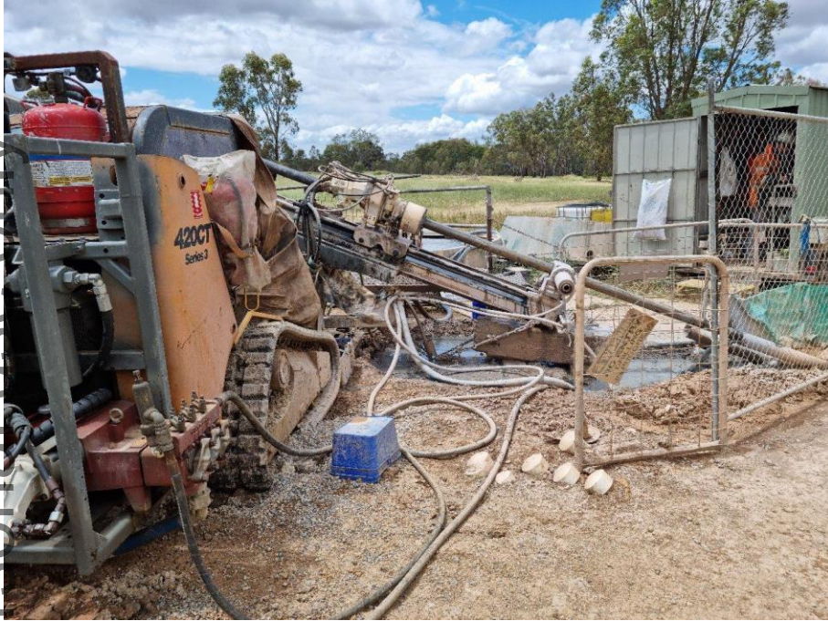
Drilling on the north side of the West Pit (NAD016 to NAD028)
