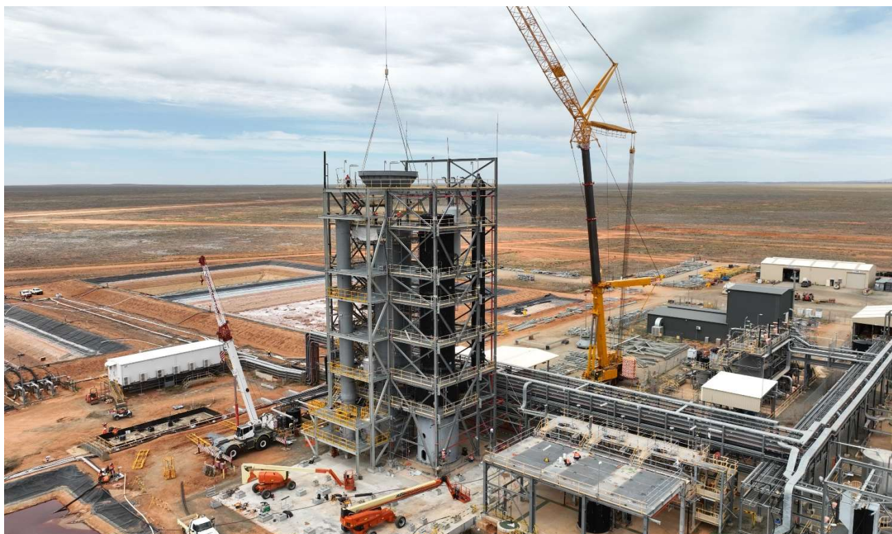
Figure 2: Installation of last section of the absorption Column 1 & steelworks
