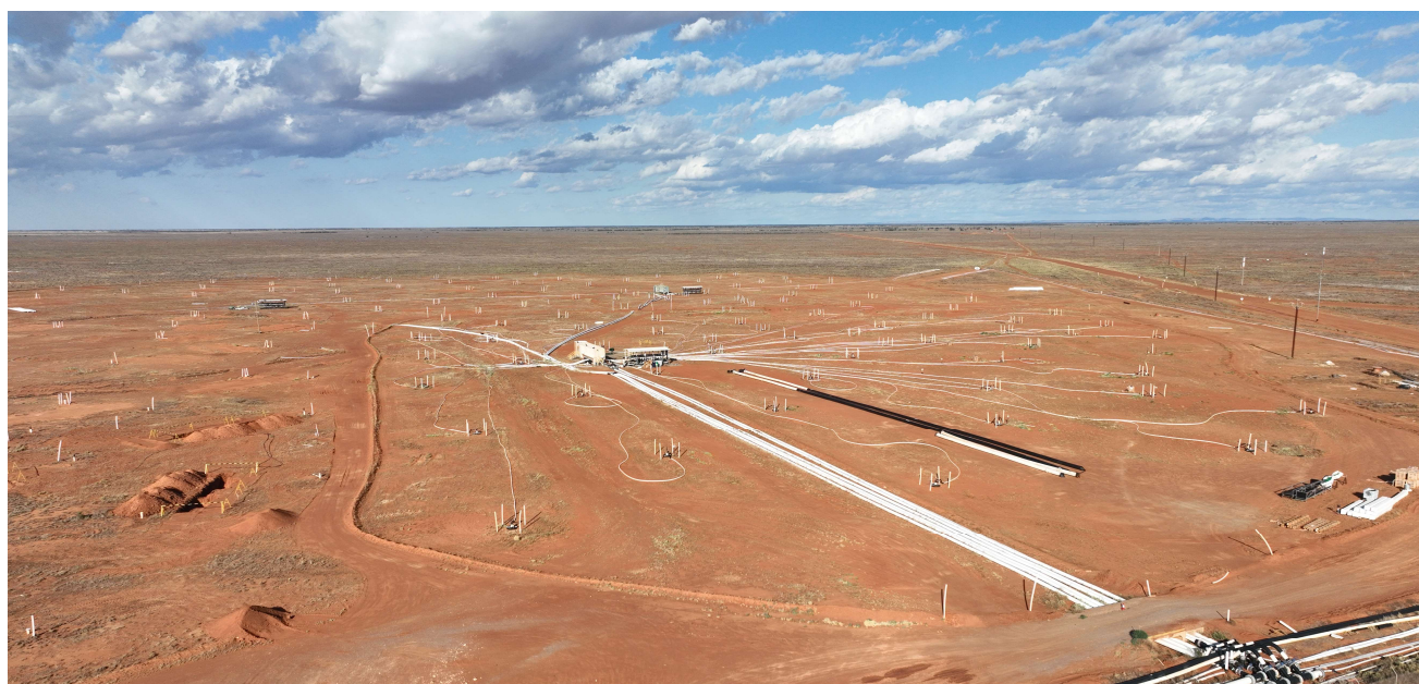
Figure 1: Pre-flushing of the Start-up Wellfields
