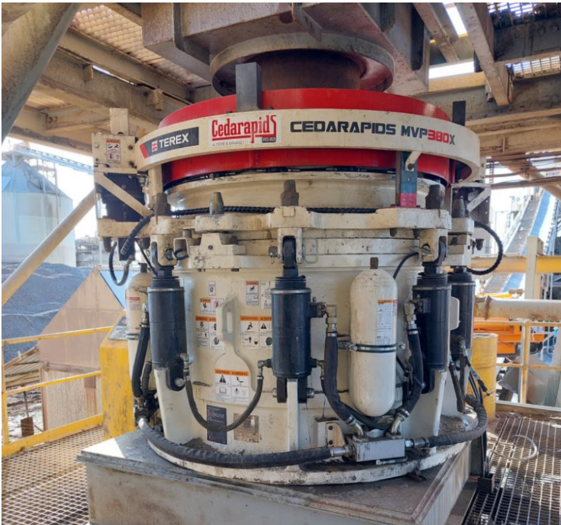
Figure 7 - New Terex 380 tertiary crusher installed
