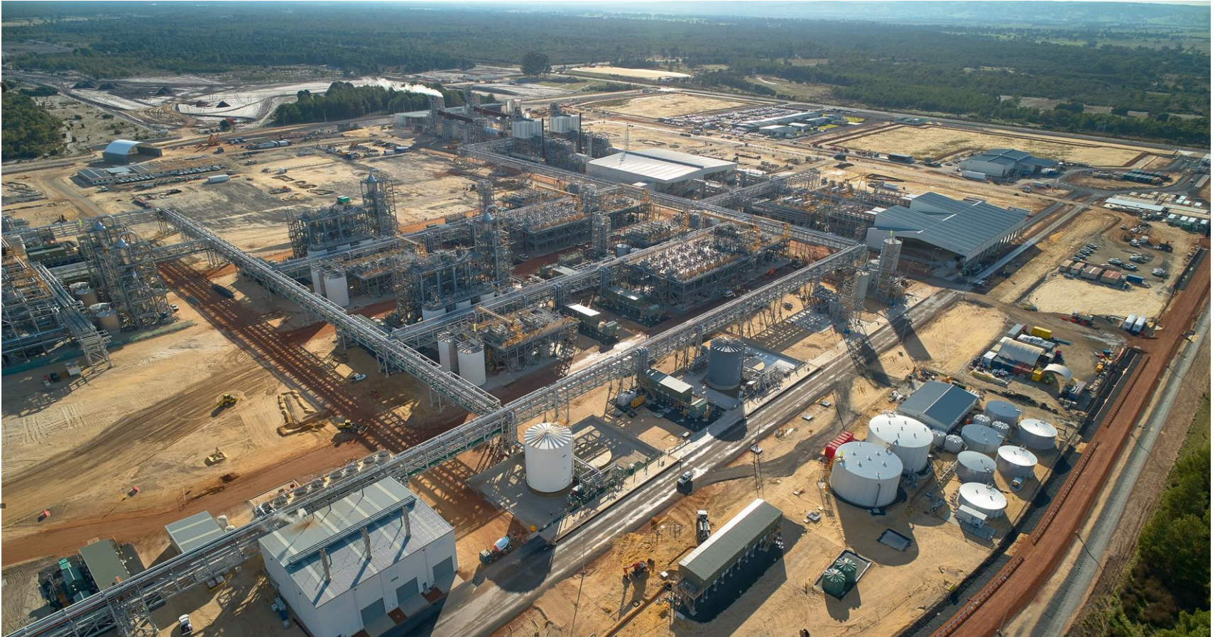
Albemarle Kemerton Lithium Hydroxide Plant, south west region, Western Australia.
