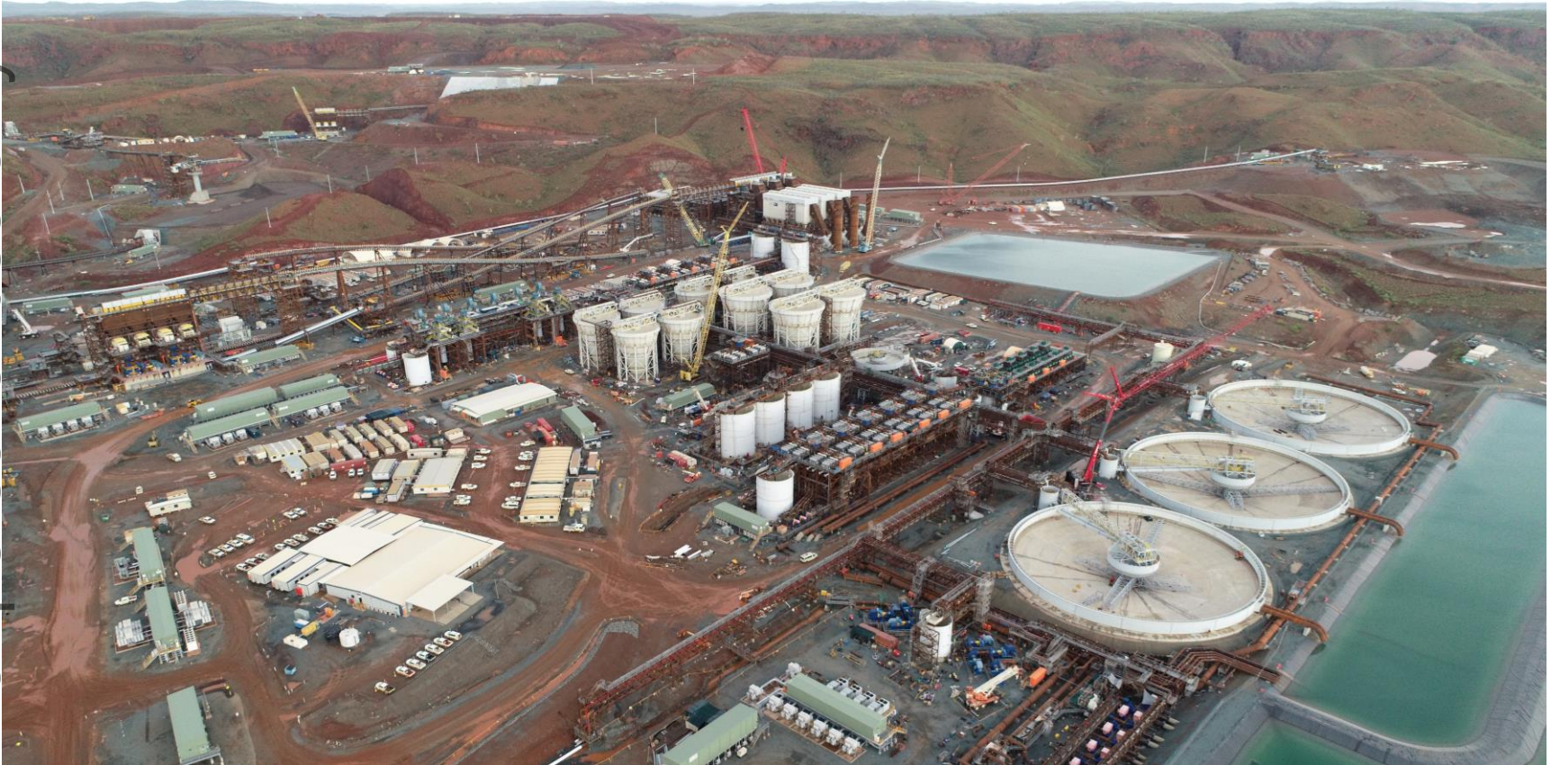
Iron Bridge Magnetite Project, Pilbara region, Western Australia.
