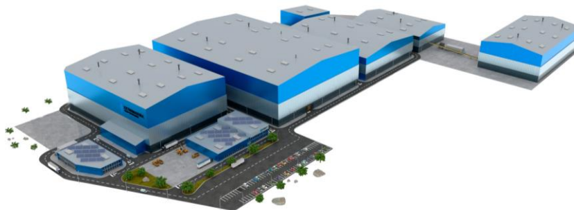
Figure 12: San José Lithium Chemical Processing Facility
