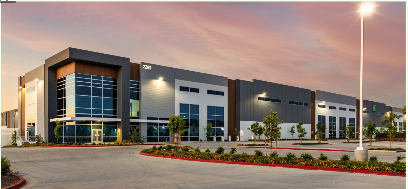
Goodman Logistics Centre, Fullerton, Los Angeles, USA.
