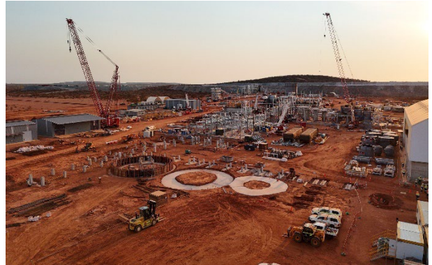
Figure 10: Process plant looking towards ROM Pad
