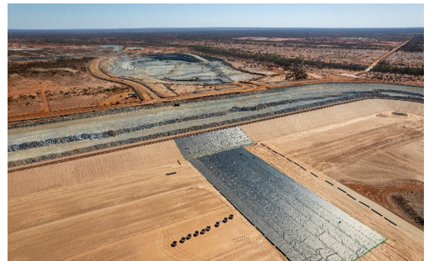
Figure 6: TSF lining in progress
