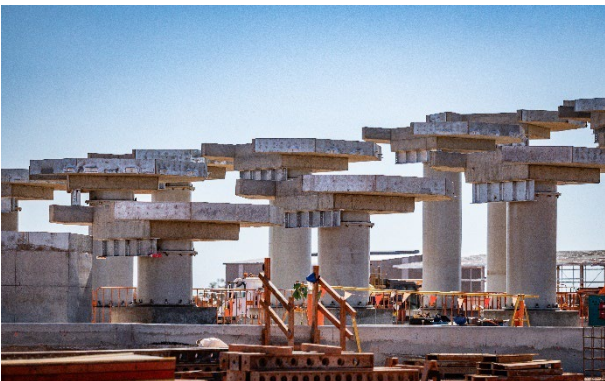
Figure 13: Flotation pedestals complete
