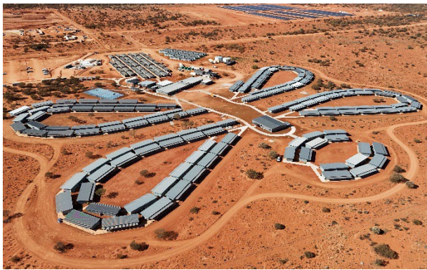
Figure 19: 676 permanent rooms installed and commissioned
