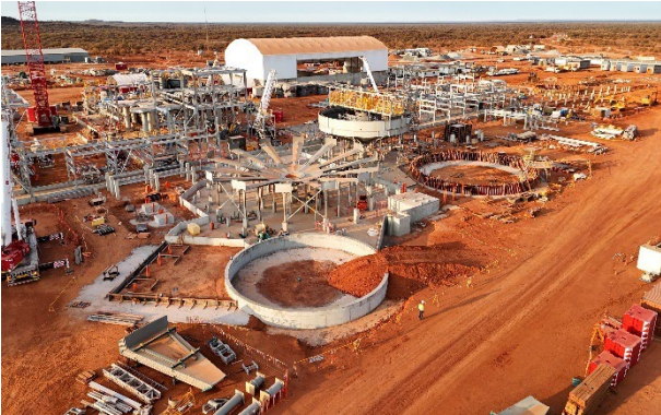
Figure 9: Progress of Wet Plant with thickening area in foreground
