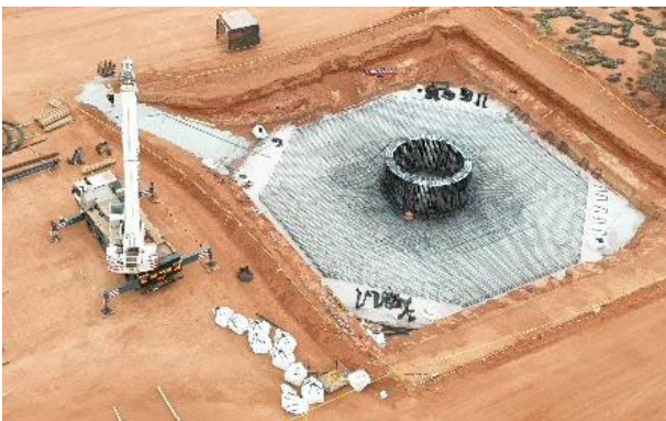
Figure 17: Aerial view of civil works at wind turbine 5
