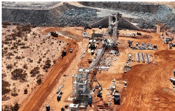
Figure 11: Progress of Dry Plant area
