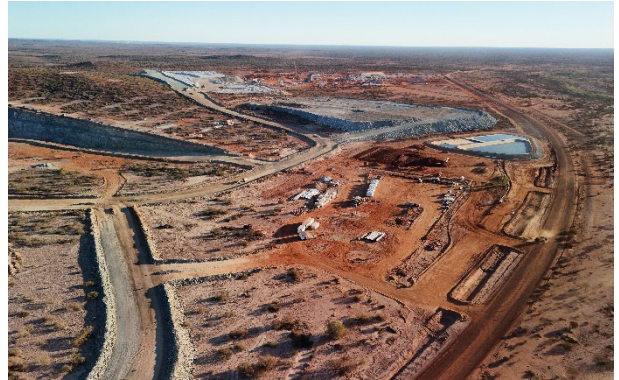
Figure 4: Aerial view of temporary U/G MSA and paste fill plant pad
