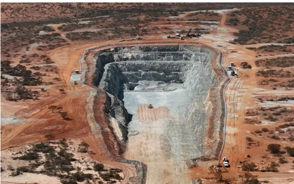
Figure 5: Preparation of Mt Mann box cut for U/G operations underway
