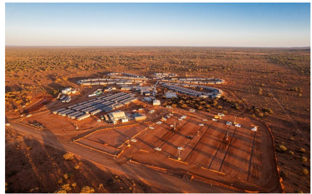
Figure 20: Camp aerial view
