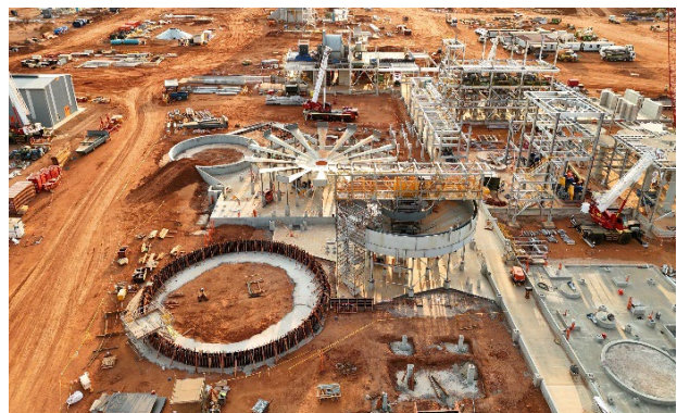
Figure 8: Process Plant concrete nearing completion
