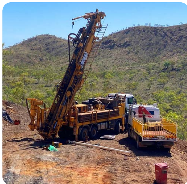
Drilling at Kalman
