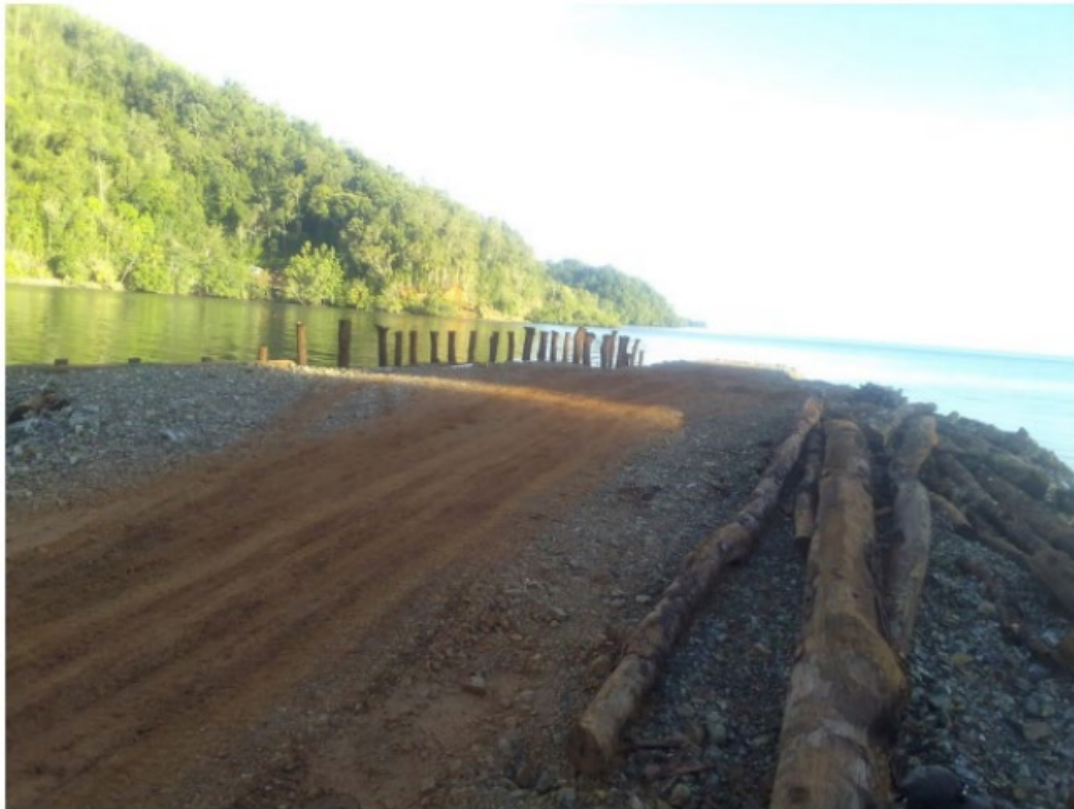
Construction of eastern face of DSO Loadout Wharf
