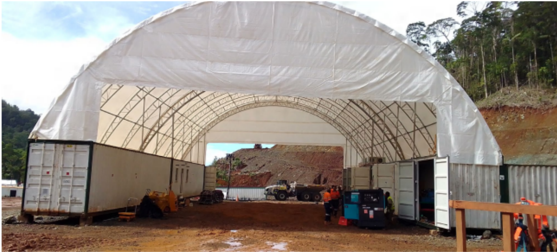
Mining contractor workshop area established
