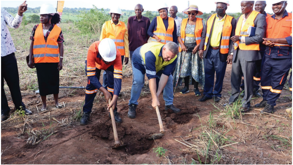
Figure 5: Makuutu Demonstration Plant ground-breaking performed by RRM Country Manager, Patience Singo (left), and Ben Vietnieks (ADT Africa, Right) along with Bugweri District officials at the Makuutu Demonstration Plant site in the Makandwa Village, Makuutu Sub-County.
