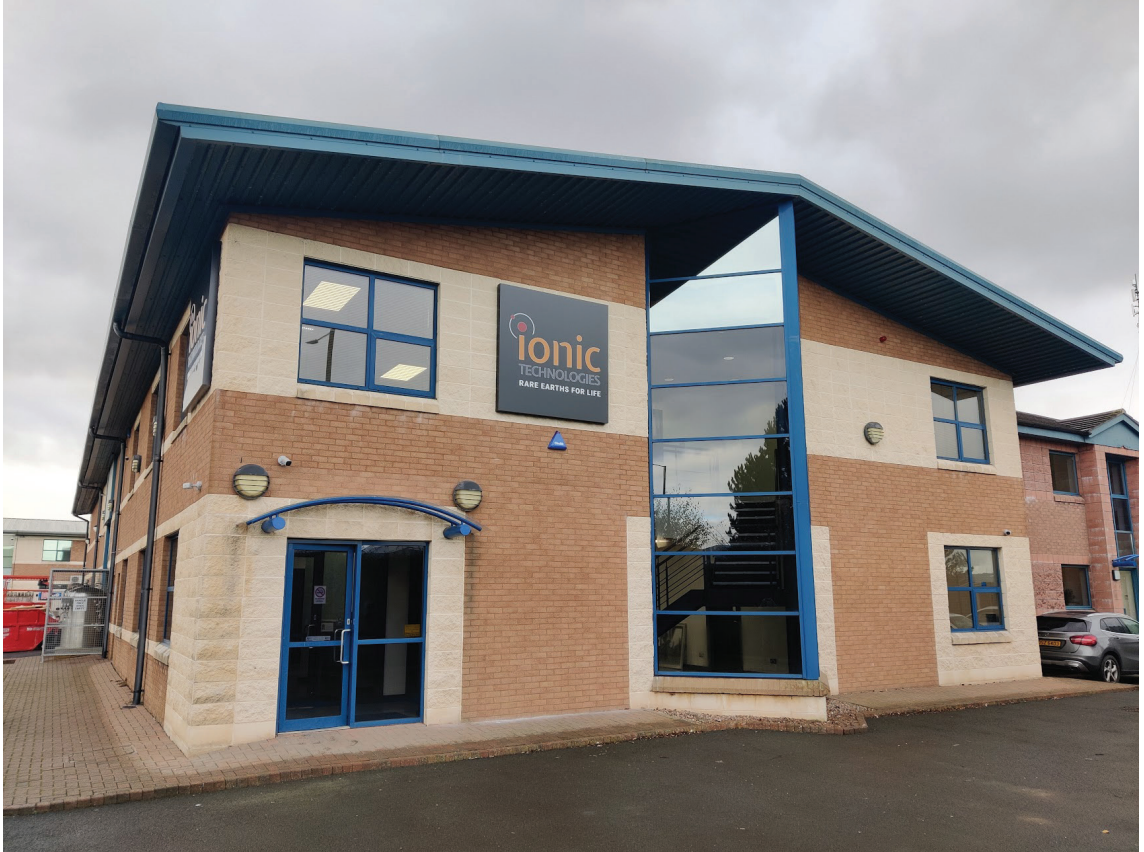
Figure 7: Ionic Technologies new facility located at the Titanic Quarter, Belfast, UK.
