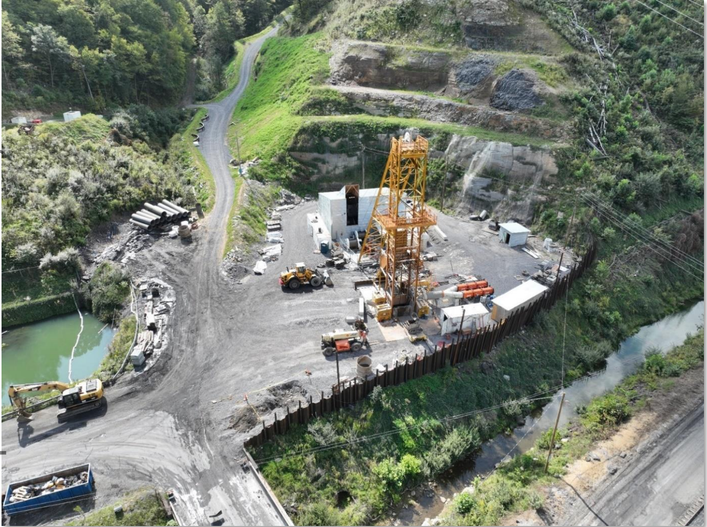
Image: Installation progressing on second set of skips – Buchanan Mine
