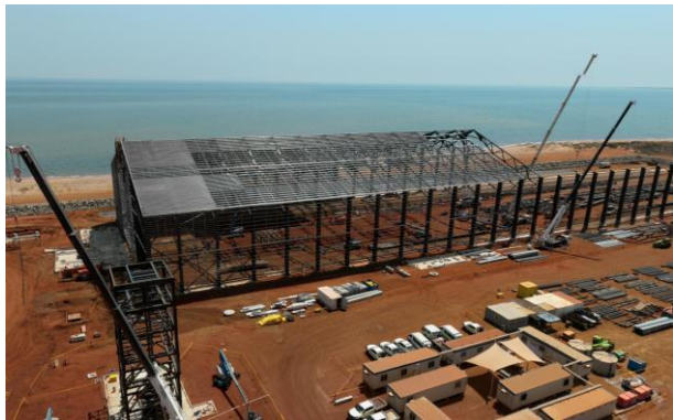
Port ore storage shed steel erection
