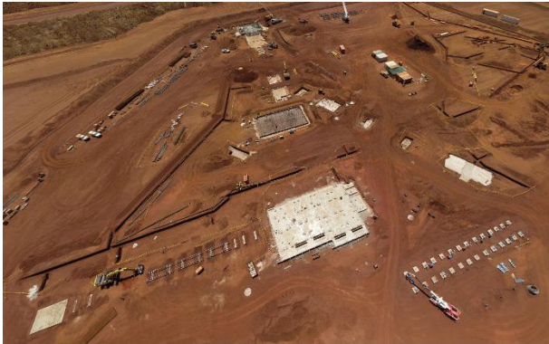
Ken's Bore crushing plant pad concrete works
