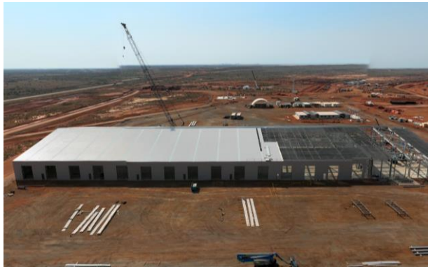
Road train truck maintenance facility
