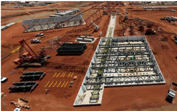
Unloading shed feeder installation
