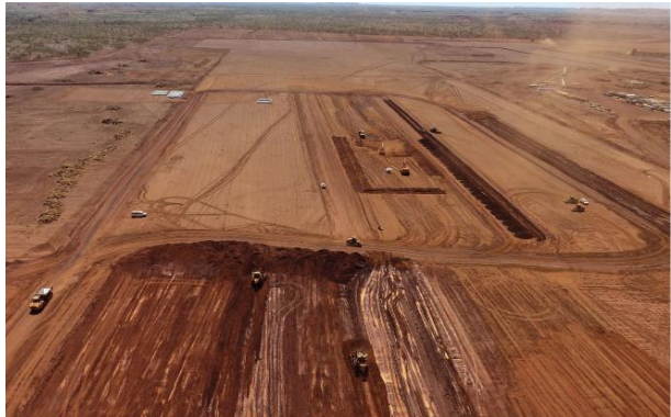
Stockyard earthworks progressing
