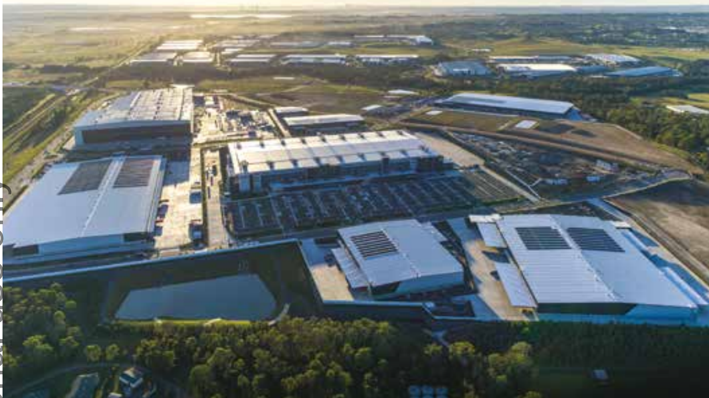
Oakdale West Industrial Estate Western Sydney, NSW
