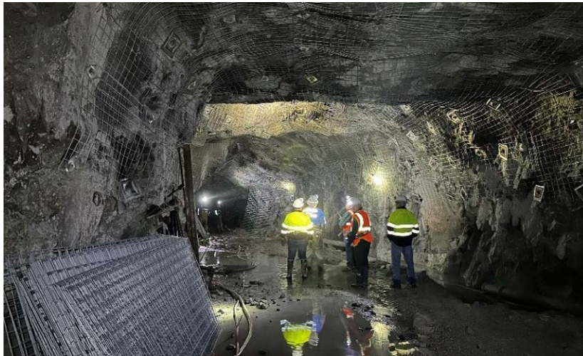
Underground mine refurbishment in progress
