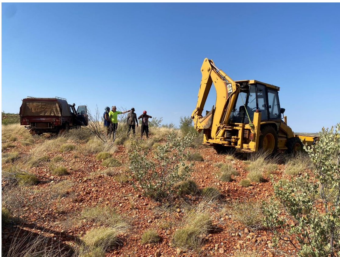
Figure 2. Site Preparation at the Webb Project
