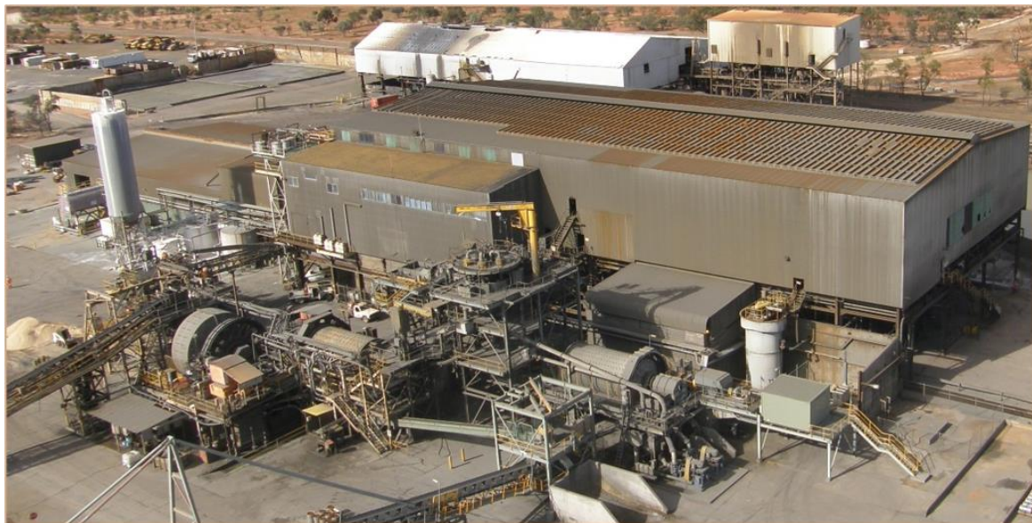
Figure 31: Endeavor Mine Processing Plant
