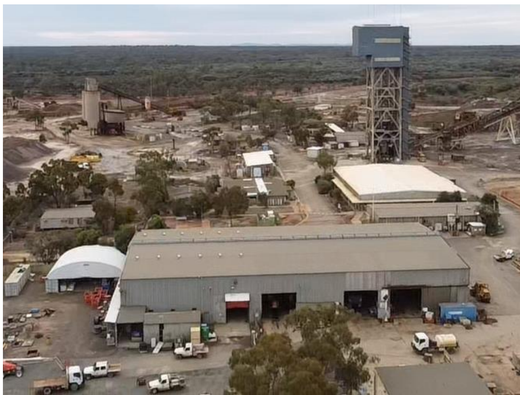
Figure 40: Workshop and Stores (foreground), Offices and Headframe
