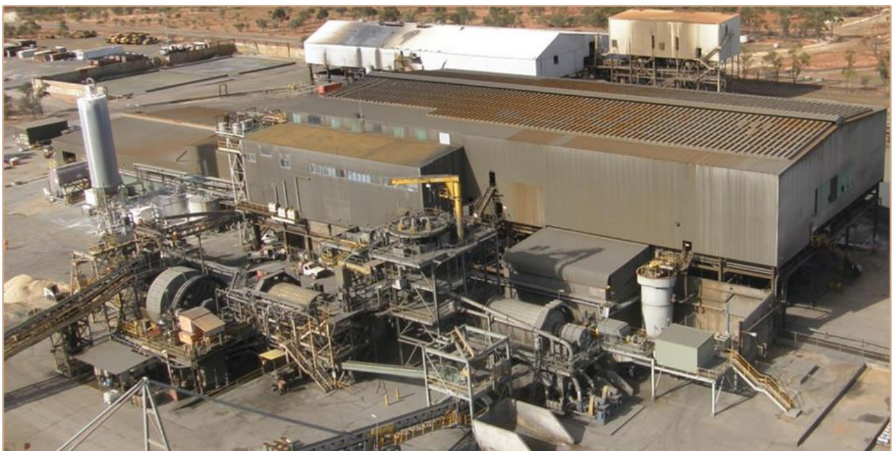
Figure 4: Endeavor Mine Processing Plant
