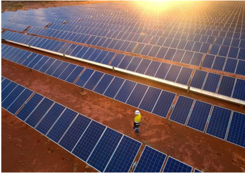
Figure 48: Example Solar Power Facility – Degrusa Mine
