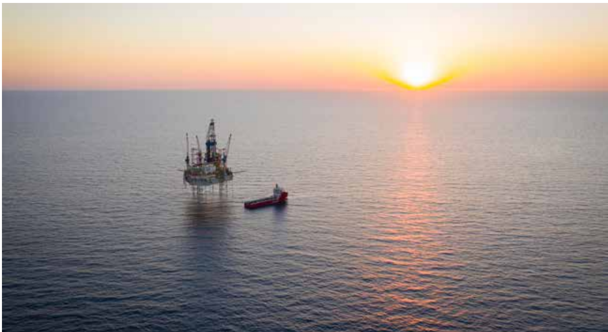
Figure 2: Image of Noble's Tom Prosser rig on site during the Dorado Appraisal campaign.
