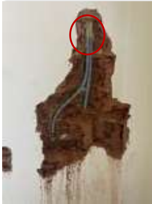
Lagging material (wrapping around pipe), which appears to be permeable – this is not compliant with the relevant Australian Standard
