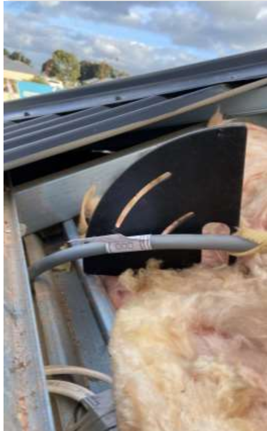
Minimum bending radius must be 10 times the outside diameter of the pipe. All of the pipes shown here have been over-bent
