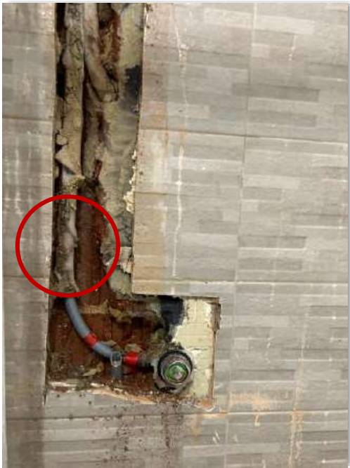
Lagging material (wrapping around pipe), which appears to be permeable – this is not compliant with the relevant Australian Standard
