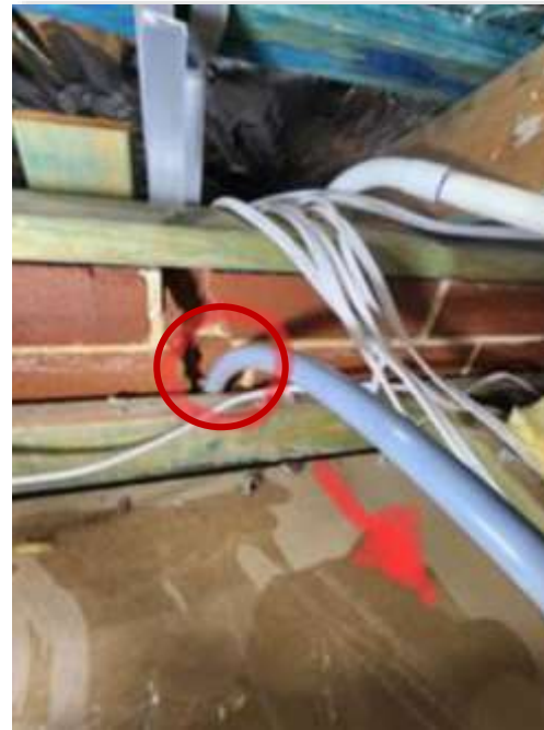
The bend of these pipes are likely to be outside of Iplex Pro-fit instructions (too tight), placing stress on the pipes
