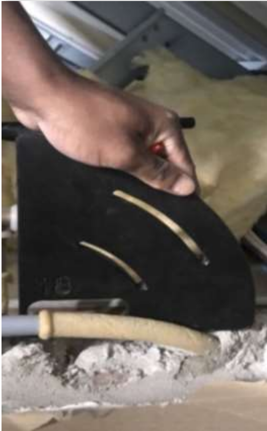
Minimum bending radius must be 10 times the outside diameter of the pipe. All of the pipes shown here have been over-bent
