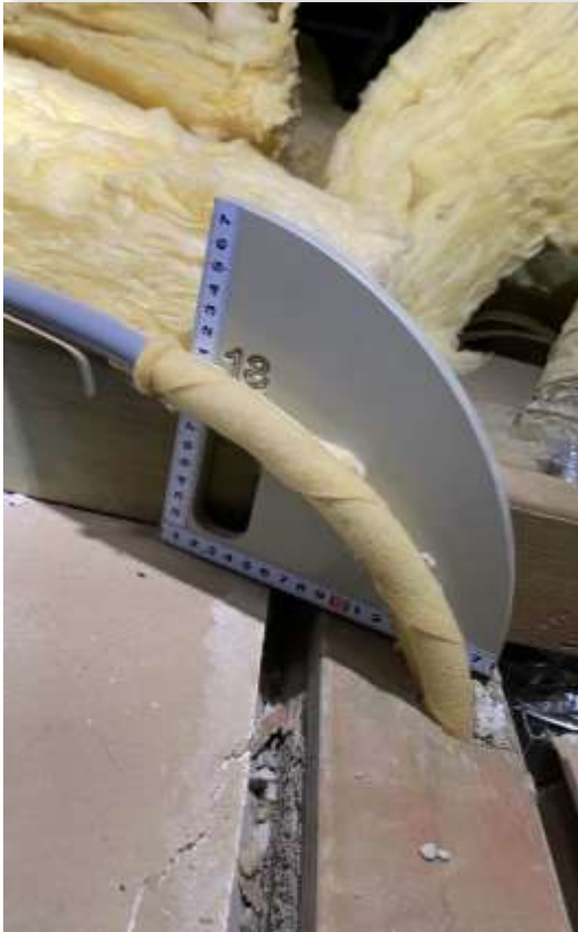
Minimum bending radius must be 10 times the outside diameter of the pipe. All of the pipes shown here have been over-bent
