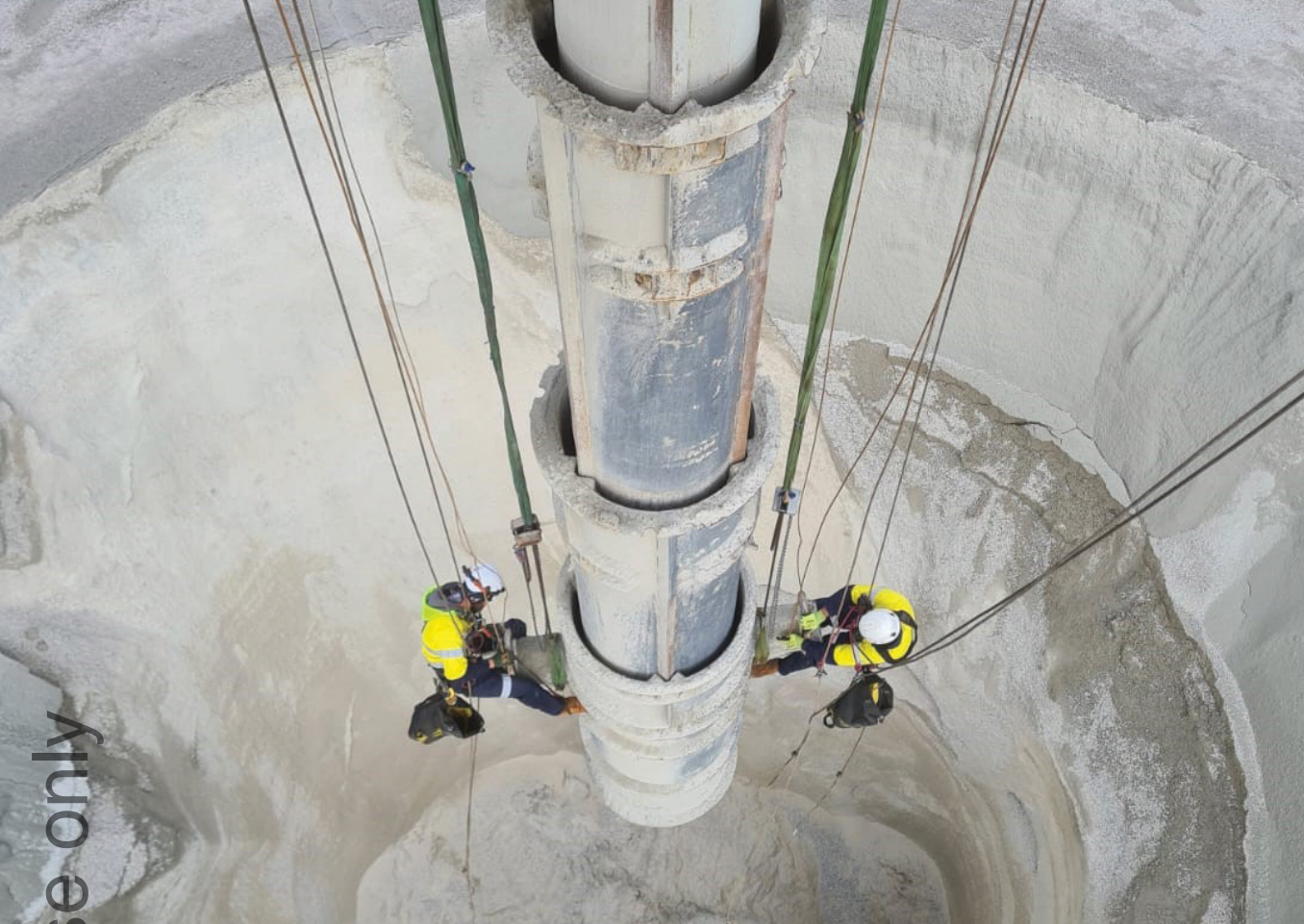
Civmec rope access crew performing maintenance
