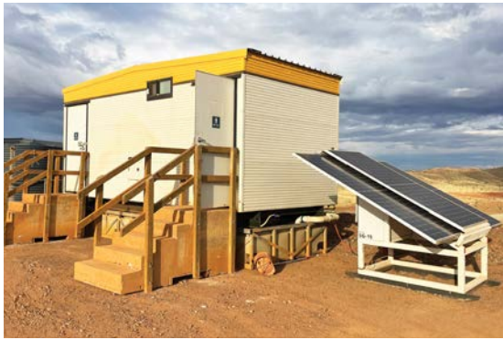
Solar and battery powered remote ablution block
