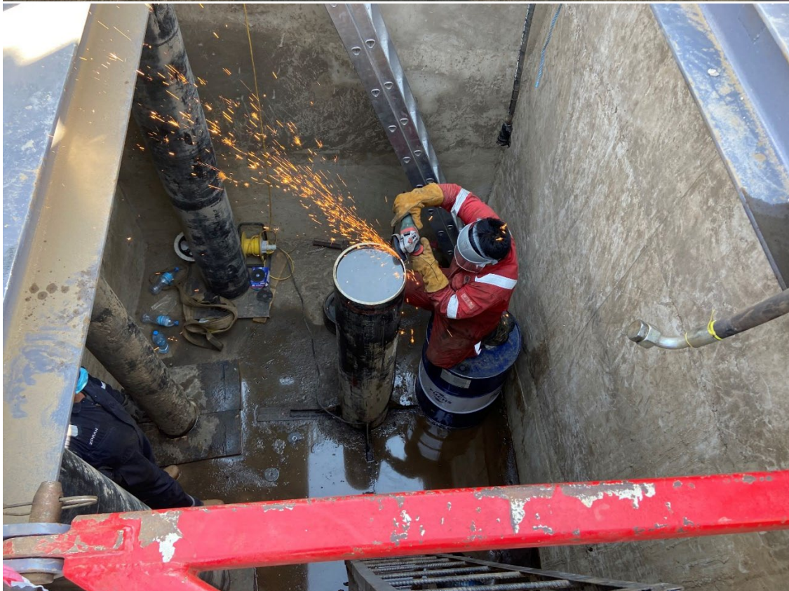
Figure 1. a) Mbelele-1 Wellsite and b) preparing for wellhead / BOP installation at Mbelele-1
